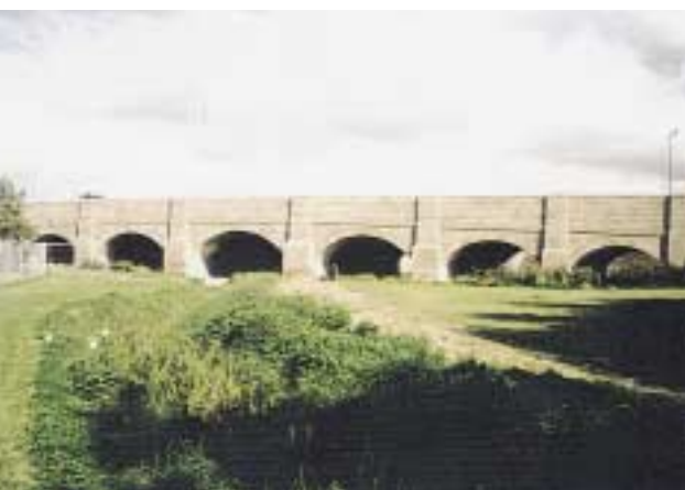
FLOOD ARCHES These arches allow passage of flood water along the flood channel of the Don at Doncaster
