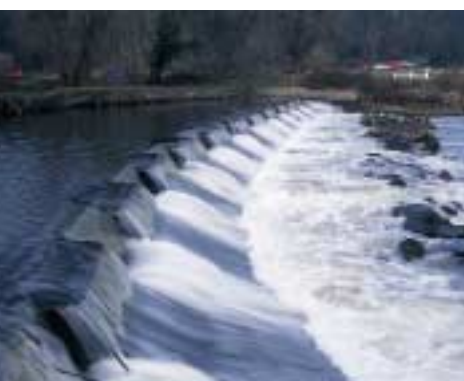
WEIR AT SPROTBOUGH The weir at Sprotbrough impounded water for two milling operations. The earliest which was used for production of flour, was built around 1279 and remained in operation well into the 20th Century
