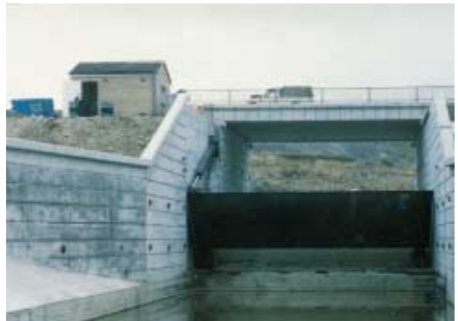
MEADOWGATE REGULATOR This regulator controls flood water on the Rother below Staveley and in extreme conditions helps to flood the washland areas which are part of the Rother Valley Country Park Complex
