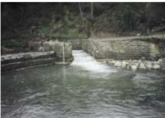
FISH PASS Current legislation demands that new obstructions or existing obstructions which are restored or rebuilt over more than 50% of their length are fitted with a fish pass
