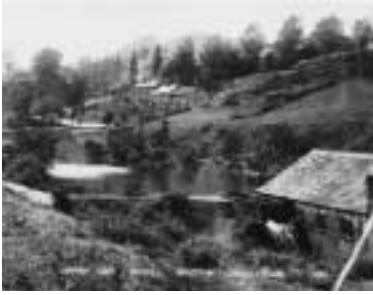
UPPER CUT WHEEL DAM ON RIVER RIVELIN A good example of the dams which were constructed to provide water to the mill of a cutlers grinding operation. The mill wheel can be seen in the foreground
