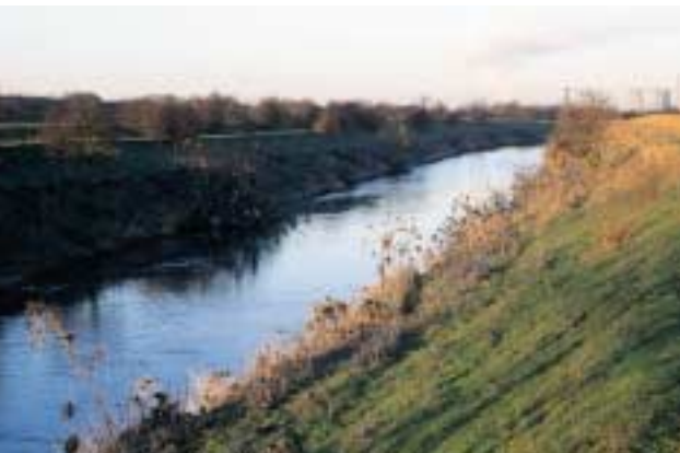
FLOOD DRAIN, DOWNSTREAM OF DONCASTER The flood drain was constructed to take excess water from the newly constructed navigation
