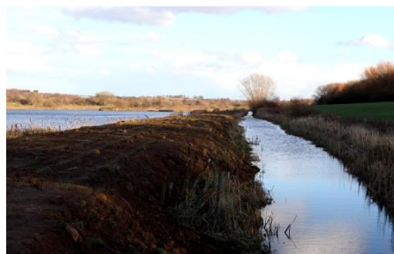
The banking before and after the works
