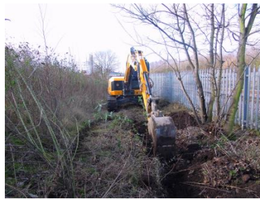
Excavation of a planting ditch
