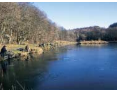
TIN MILL DAM
