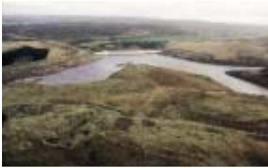
WINSCAR RESERVOIR Built to replace the smaller Dunford Bridge Reservoir in the 1970's. It serves as a compensation reservoir which provides the base flow to the upper River Don
