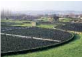
LUNDWOOD STW The main sewage treatment works for Barnsley continues to have a serious detrimental effect on water quality. An improvement scheme which commenced in 1996 should result in a significant improvement in water quality in the Dearne downstream of the town
