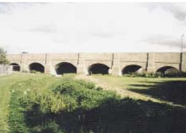
FLOOD ARCHES These arches allow passage of flood water along the flood channel of the Don at Doncaster
