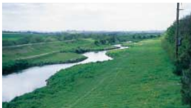
PASTURES ROAD - BEFORE AND AFTER
