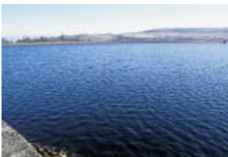
REDMIRE'S MIDDLE RESERVOIR The first large reservoir built on the Don system to provide water for drinking and industrial purposes constructed in 1830
