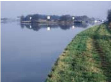
CONFLUENCE OF NEW JUNCTION AND STAINFORTH/KEADBY CANALS The beginning of the New Junction & Stainforth & Keadby Navigations at Kirk Bramwith. The entrance to the New Junction Canal is on the left of the picture.
