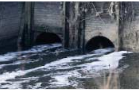
DISCHARGE FROM BLACKBURN MEADOWS STW Serving the city of Sheffield, it is the largest STW in the Don catchment
