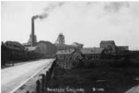
BENTLEY COLLIERY This and other collieries in the Doncaster area was responsible for subsidence problems in the land adjacent to the River Don.
