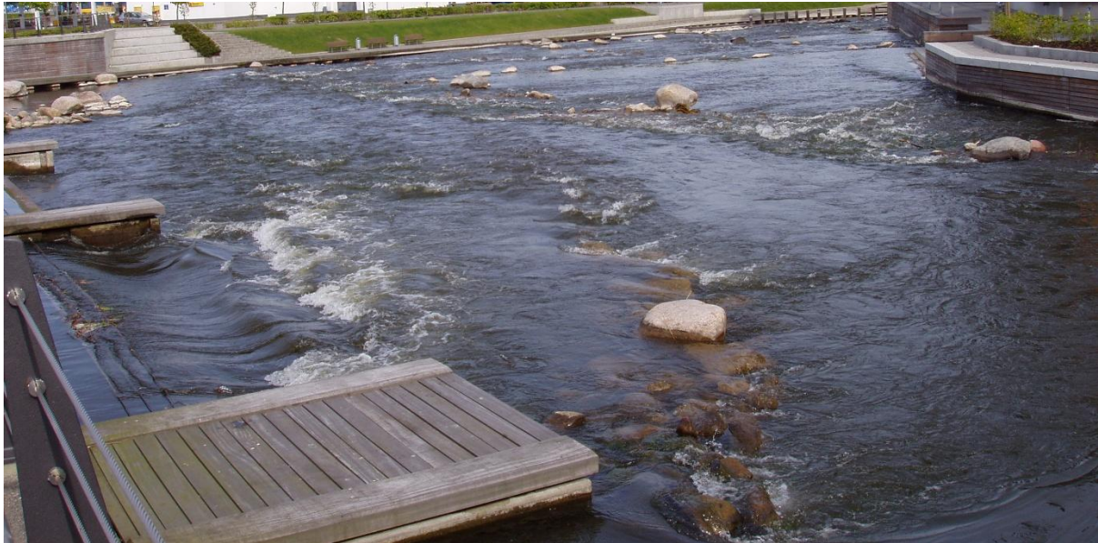
Figure 11: The step remaining at the weir crest is visible between the wooden platforms (lower left of frame). The installed easement measures do not extend to that crest, meaning an obstruction to fish passage remains at this point along the crest of the weir.
