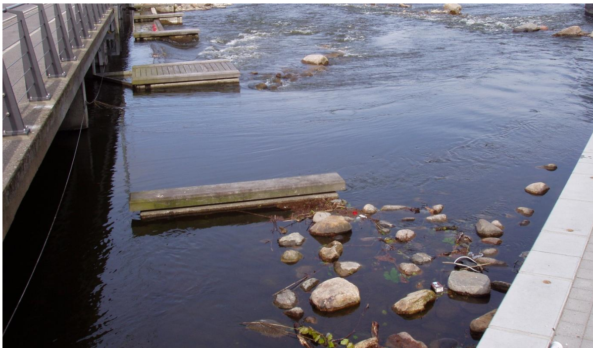
Figure 12: Slot cut into the crest (lower edge of the frame) with installed boulder cluster ensuring slot is drowned out while maintaining low flow velocity through the slot.
