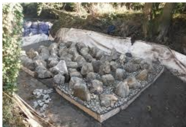
Figure 8 (construction phase): The embedded design under construction, showing dressing with smaller-diameter substrate around the base of each large boulder.
