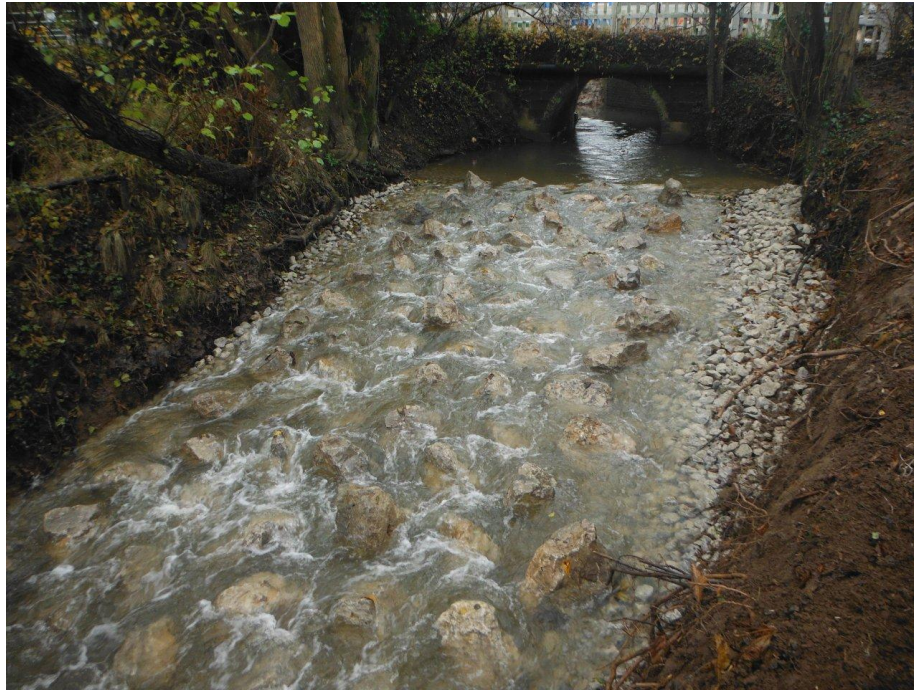
Figure 9 (completed installation): The high placement density of perturbation boulders is clearly visible. The crest of the obstacle appears well drowned out and there is a sufficient depth of water throughout the upstream culvert.
