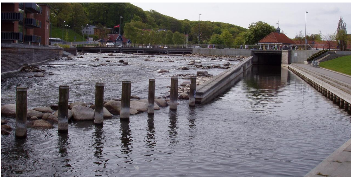
Figure 10: : Good use of channel width to minimise path-length gradient, with robust construction methods.
